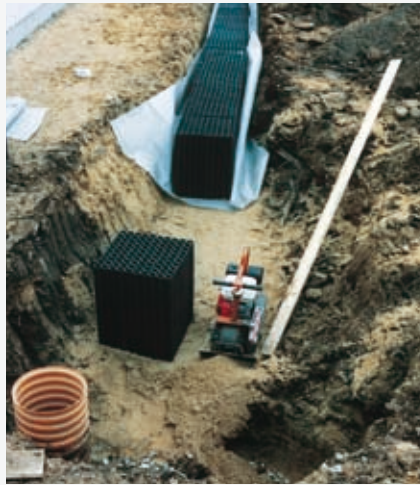
Longitudinal drywell, industrial area
