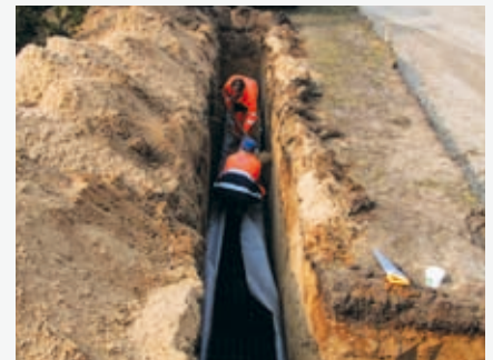
Drywell being installed
